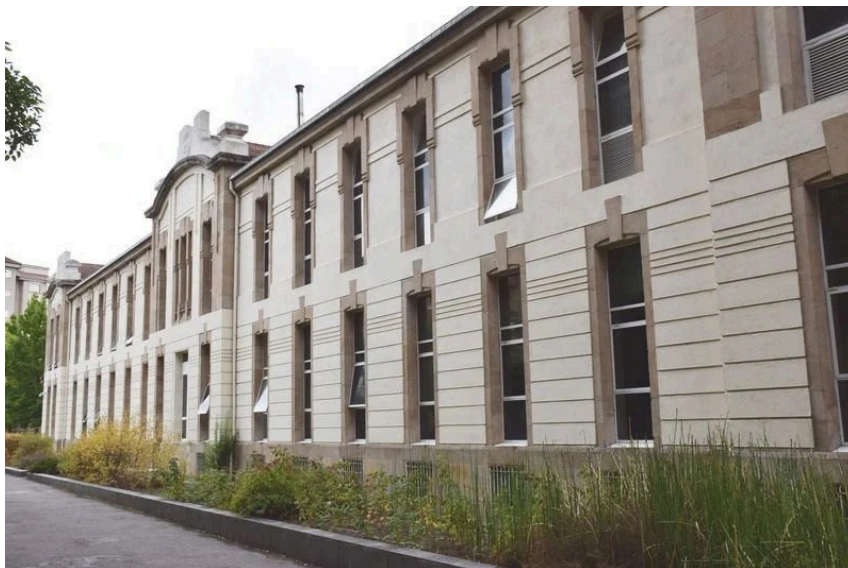
Figure 1. Building of the Institute of Physics and Aerospace Sciences (IFCAE) at Ourense, Spain.
